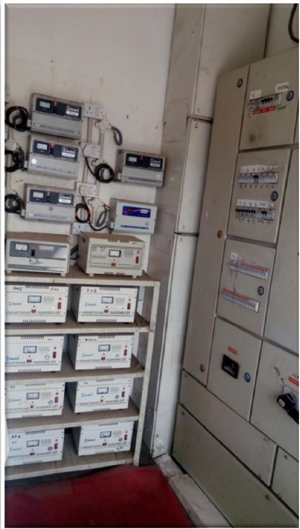
Before Installation of TSi-VRP
